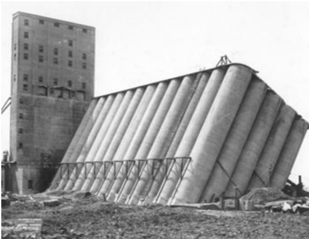
Failure of Transcona Grain Elevator
