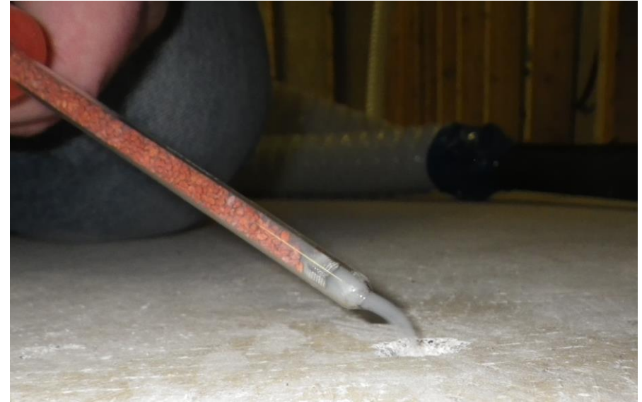
Negative pressure under the slab
